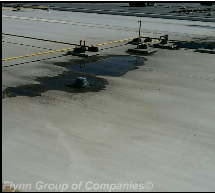
Section_B: Drain in need of cleaning.
