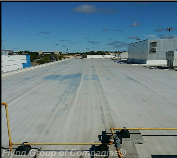
Section_B: View east on section_b.
