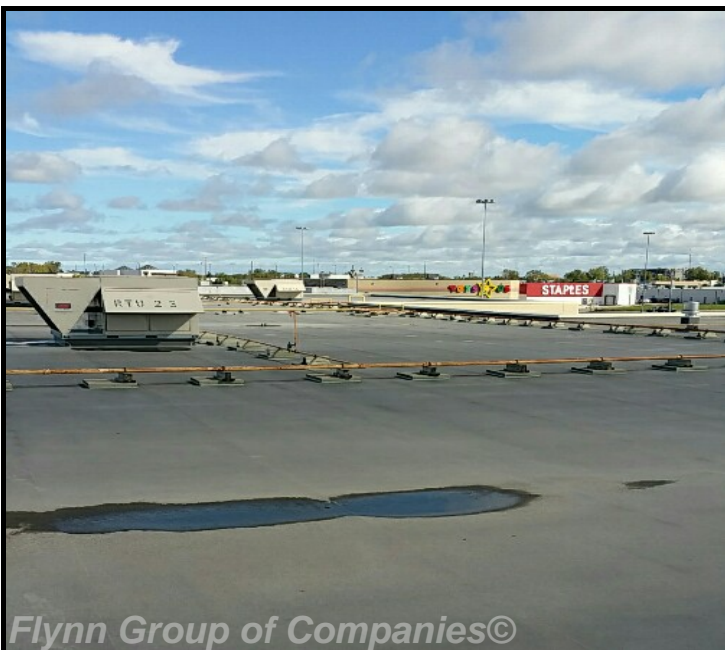
Section_A: Overview of roof section A looking north.
