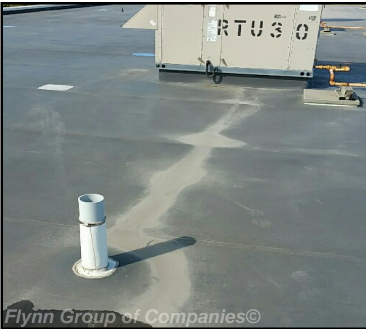
Section_A: Field fabricated pipe boot
