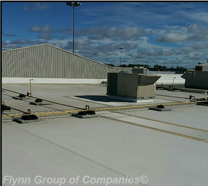
Section_B: backside of parapet wall .
