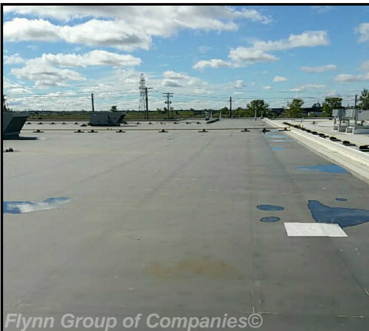
Section_A: view looking west
