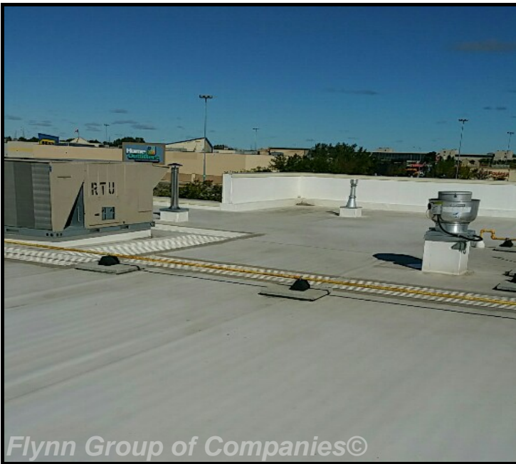
Section_B: Parapet wall, grease vent and unit on section_b.
