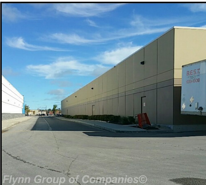
Overview: Exterior view of the south side of the building.
